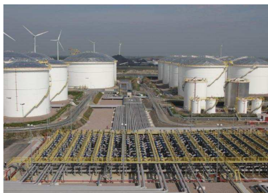
View on the central manifold.
